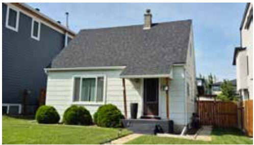
Presumed Wartime Housing Limited dwelling at 1823-31 Avenue SW, photographed July 17, 2025. Bob van Wegen, photographer.
