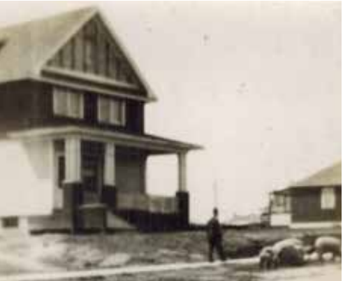
Possibly the house at 1620–33 Avenue SW, home of Eveline & Ernest Fockerd and Ada & Robert Gordon Eakin, n.d.
