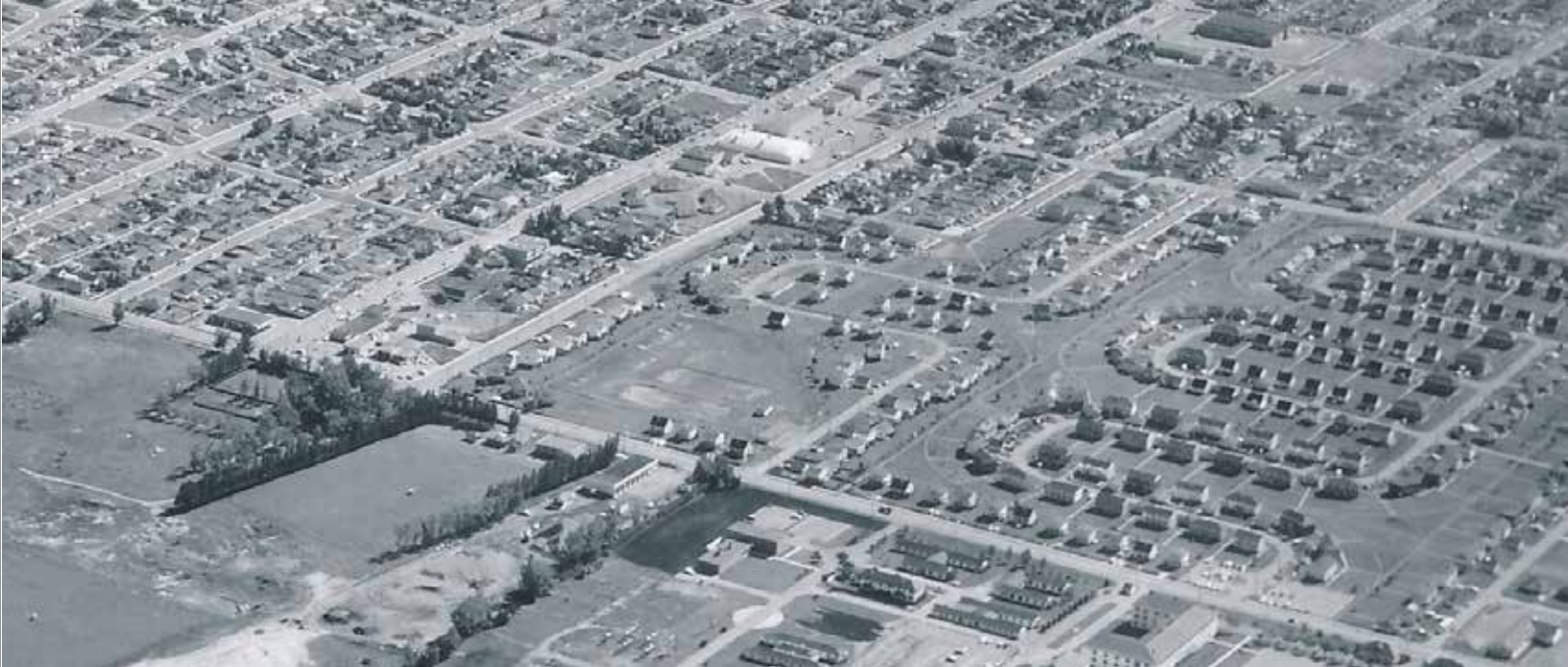
Oblique aerial view of Currie Barracks (foreground), the Currie PMQs (above right), and the 33 Avenue SW business district west from 20 Street SW, 1963.
