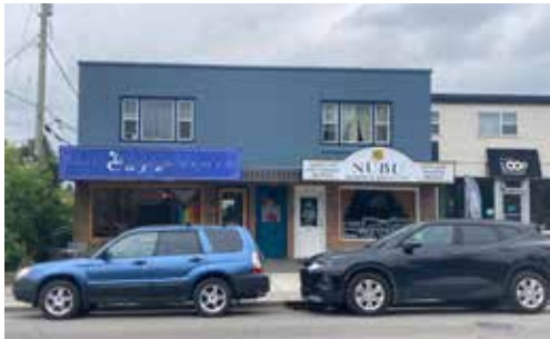
Harold Garfield (Buzz) McKittrick constructed the building at 1515-34 Avenue SW in 1953, and it housed McKittrick Hardware for many years. in name and logo.
