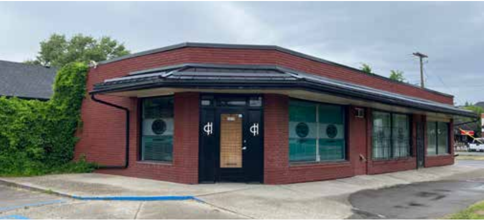
Commercial building at 2911, 2913, 2915–14 Street SW, June 30, 2024. Wilfred F. Costello had this building constructed in 1954.
