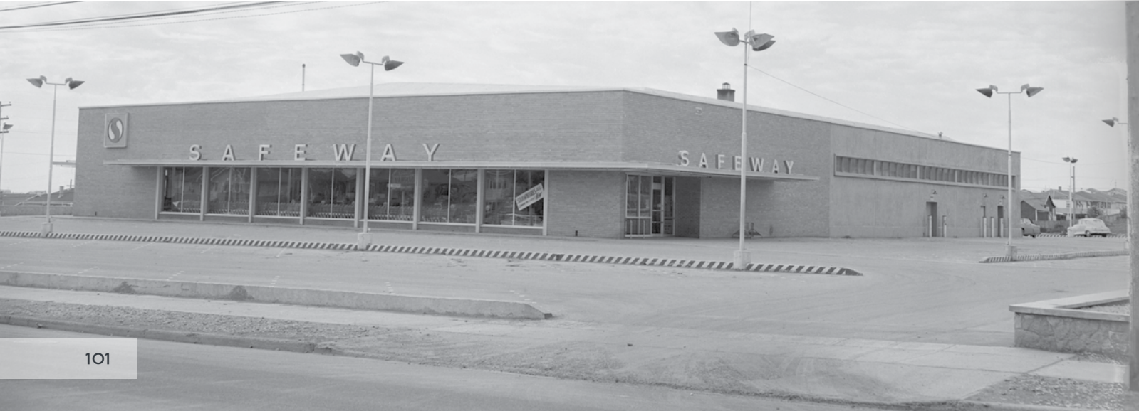
Altadore Safeway (1811–34 Avenue SW), 1957. The store was built in 1955 and demolished around 2000.
