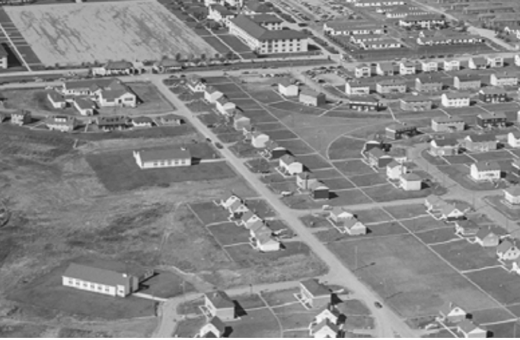
This undated photograph, looking west, shows the relative positions of Currie Barracks, the former Salvation Army Red Shield Hut, and the two chapels built in the Currie PMQs in 1956. The gates of Currie Barracks are visible at the top centre. The J-shaped former Red Shield Hut is shown on the near side of 24 Street SW (the future Crowchild Trail) from the barracks gates. The Chapel of St. George, centre, is shown fronting Cambrai Avenue SW, the road leading east across 24 Street SW from the barracks gates. Christ the King Chapel can be seen in the left foreground. C.N. Ross, photographer.
