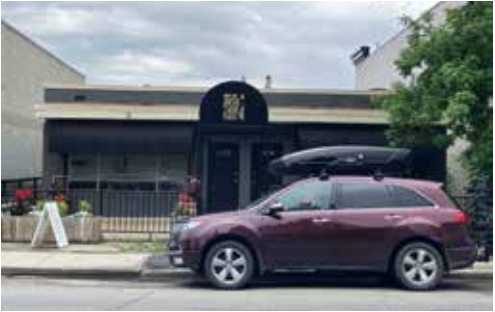
Wilfrid F. Costello built the extant commercial building at 4018, 4020–16 Avenue SW in 1951. Photographed on June 18, 2024.
