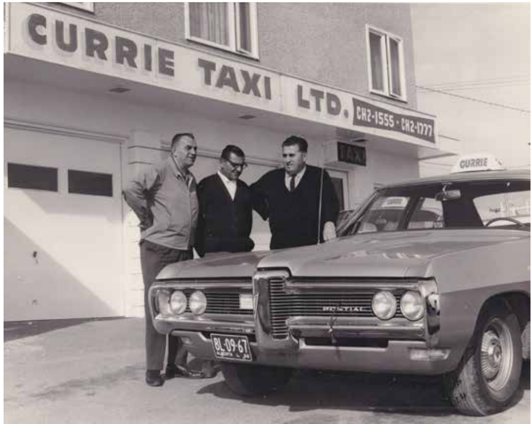
Looking northwest toward the east facade of Currie Taxi (2442–34 Avenue SW), circa 1968. The building remains extant as Mike’s Auto Service.
