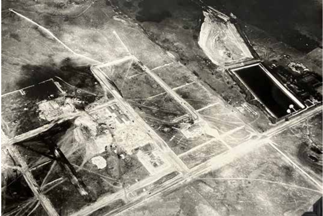
Oblique aerial view of Currie Barracks construction, looking northwest, July 25, 1935. A corner of the future Currie Permanent Married Quarters, which eventually became Garrison Woods, appears in the lower right corner. The road separating this area from Currie Barracks (left) and the South Calgary Reservoir (right) is 24 Street SW, the future Crowchild Trail.
