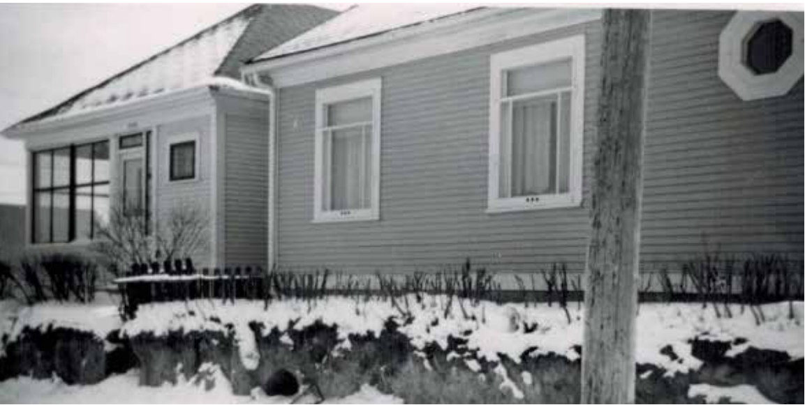
Fockerd residence (1707–34 Avenue SW), 1955.
