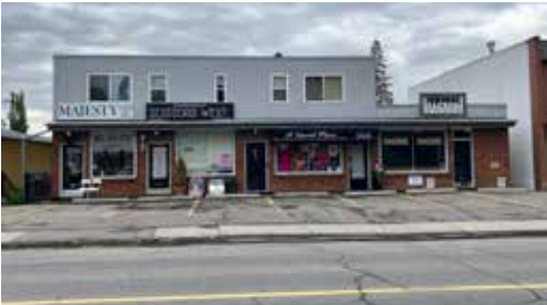
R.A. Lomow built the extant commercial building at 4004 to 4008–16 Street SW in 1955. Photographed on June 18, 2024.
